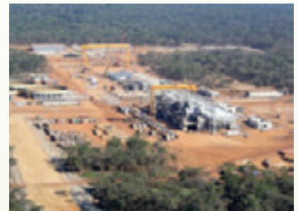
View of Kalumbila Mine in Zambia
